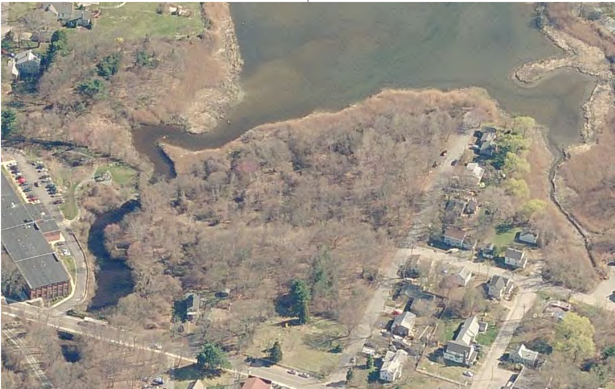
Figure 2: This undeveloped parcel on Bay Spring Avenue abutting Allin's Cove is the last Limited Manufacturing-zoned area in town. (A portion of the property is zoned Residence I0.) The site abuts Allin's Cove, classified by CRMC as Type I Conservation Waters, a designation that carries the strictest requirements for setbacks and buffer zones, and prohibits any discharges.
