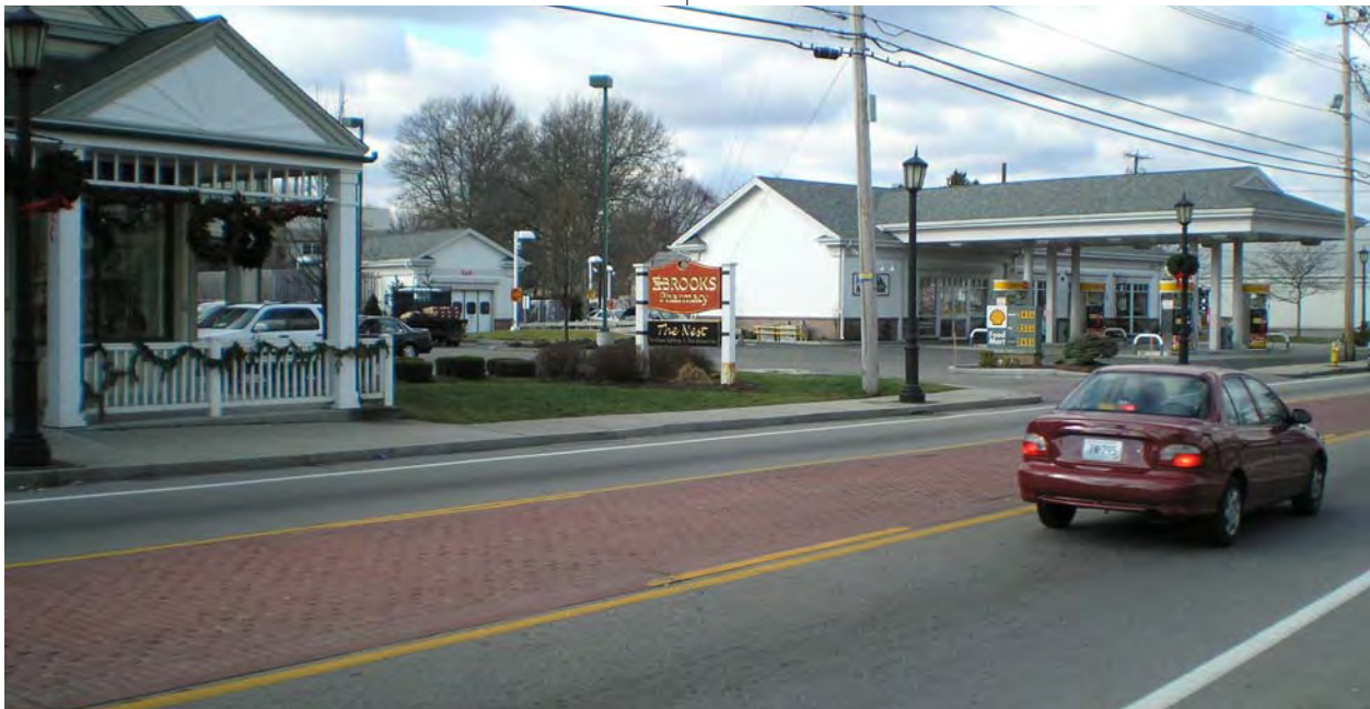
>Photo: Streetscape improvements completed in 2000 on County Road included new curbing, street lights and a "brick" center turn lane. Overhead utility lines were not placed underground due to cost.
