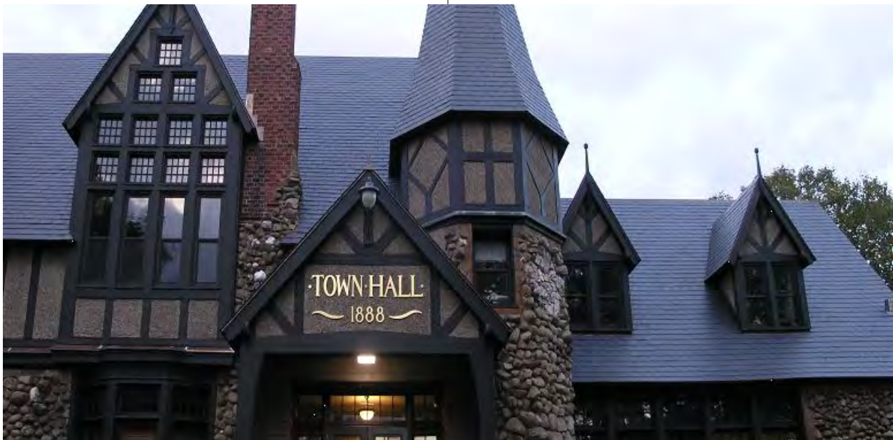
> Photo: Barrington's historic Town Hall received a new slate roof and updated exterior paint as part of historically-sensitive renovations completed in 2006.
