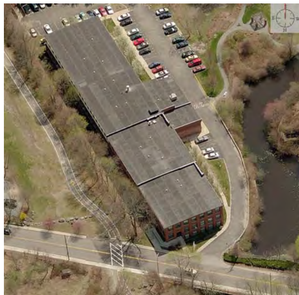
Figure 3: O'Bannon Mill (now Barrington Cove Apts)
