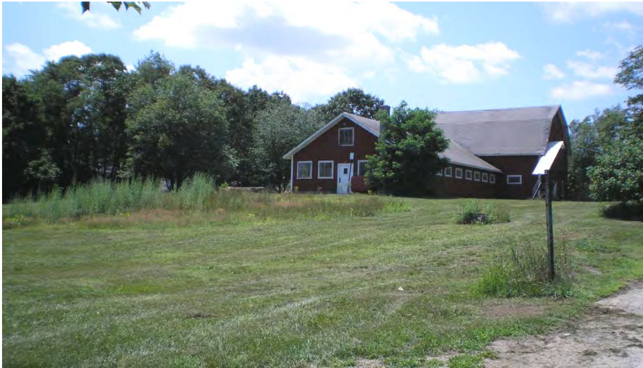
Figure 2: The building that once housed “The Place” teen center was demolished in 2007 due to structural concerns. The 5-acre site is now vacant.
