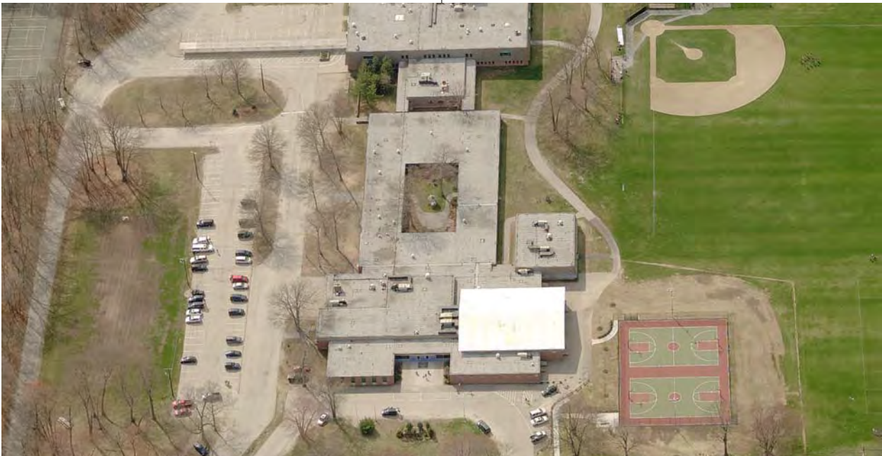
Figure 4. Schools, such as the Middle School above, are opportunities to install energy efficiency improvements and renewable energy technology.
